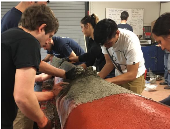
Figure 18: Structural Mix Placement
